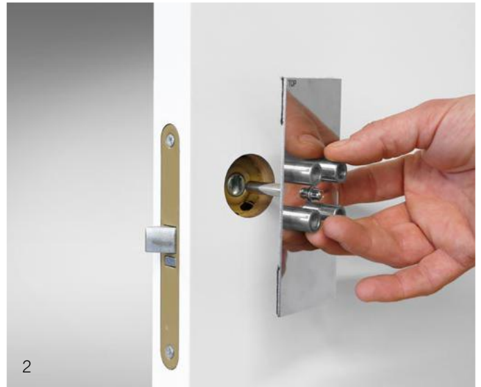
Image 2 Inserting the drilling template for lock "Boda".
