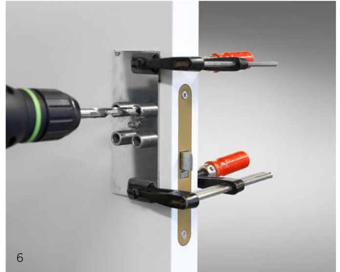
Image 6 Drilling from the lefthand side of the door. Drill through the top righthand bushing on the drilling template. Important: do not drill into the lock case.
