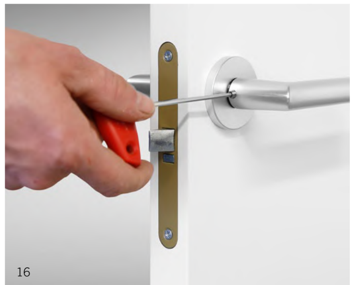
Image 16 Use an Allen key to tighten the righthand grub screw.
