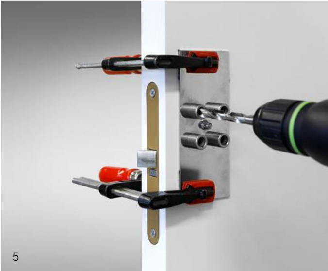
Image 5 Drilling from the righthand side of the door. Drill through the top lefthand bushing on the drilling template. Important: do not drill into the lock case.
