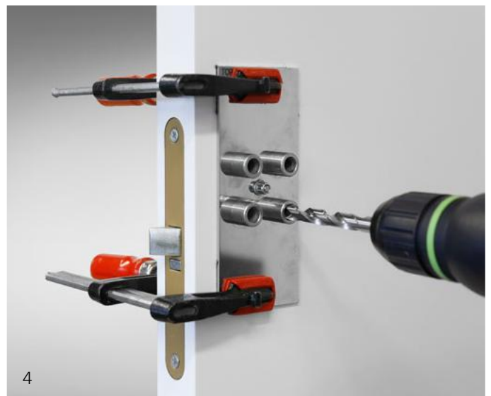
Image 4 Drilling from the righthand side of the door. Drill through the bottom righthand bushing on the drilling template. Important: do not drill into the lock case.
