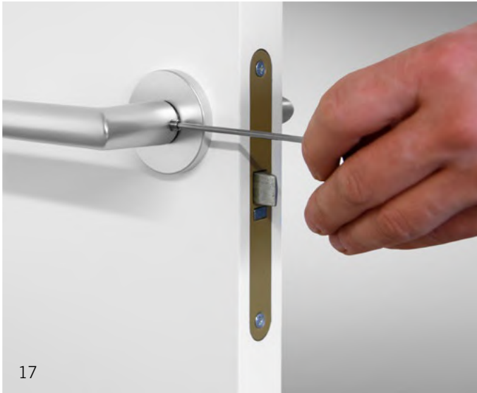
Image 17 Use an Allen key to tighten the lefthand grub screw.
