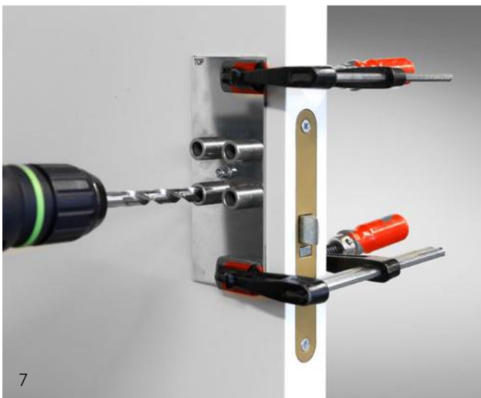
Image 7 Drilling from the lefthand side of the door. Drill through the bottom lefthand bushing on the drilling template. Important: do not drill into the lock case.
