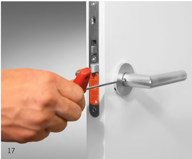
Image 17 Use an Allen key to tighten the righthand grub screw.
