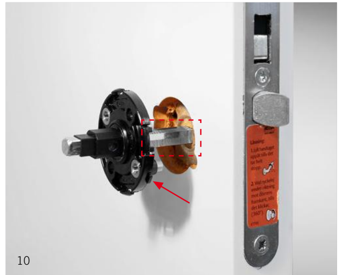
Image 10 Fitting the spindle from the lefthand side of the door. Make a careful note of the position of the notch; cf. area marked in red in the figure. Slot on the FSB ASL ® baserose, pointing it in the direction of the forend as shown.
