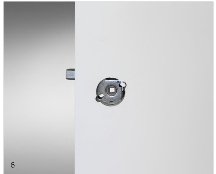
Image 6 Completed boreholes on the righthand side of the door.
