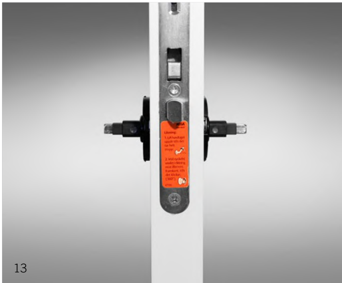
Image 13 Ensure the spindle is positioned centrally.
