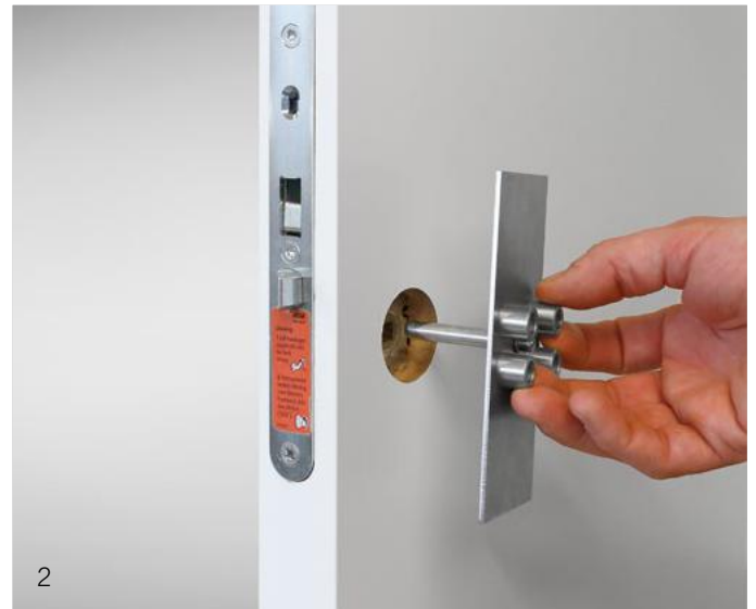
Image 2 Inserting the drilling template for lock "Assa".
