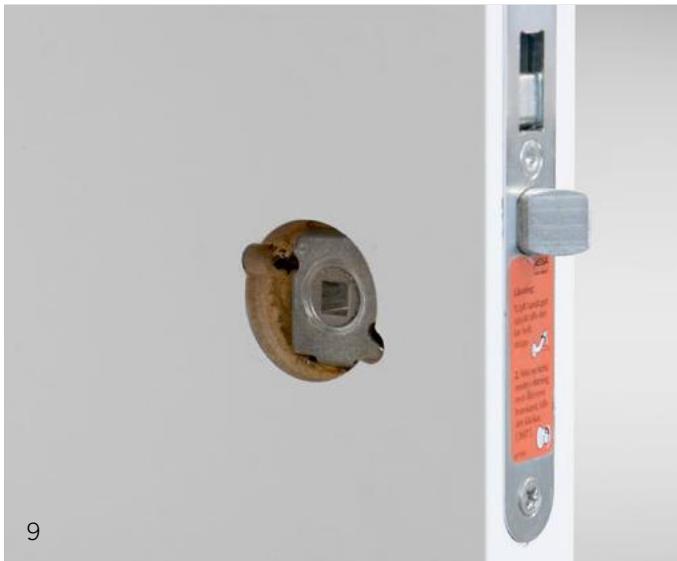
Image 9 Completed boreholes on the lefthand side of the door.
