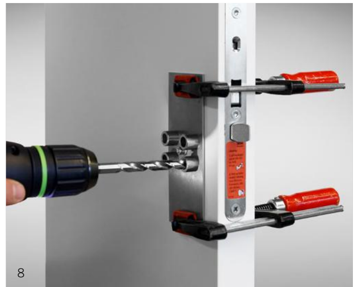
Image 8 Drilling from the lefthand side of the door. Drill through the bottom righthand bushing on the drilling template. Important: do not drill into the lock case.
