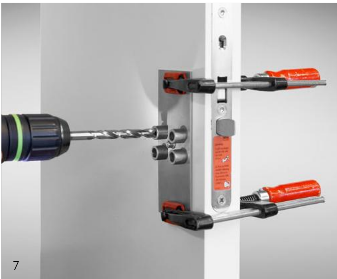
Image 7 Drilling from the lefthand side of the door. Drill through the top lefthand bushing on the drilling template. Important: do not drill into the lock case.
