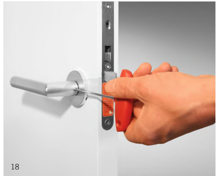
Image 18 Use an Allen key to tighten the lefthand grub screw.
