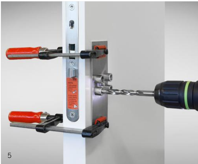
Image 5 Drilling from the righthand side of the door. Drill through the bottom lefthand bushing on the drilling template. Important: do not drill into the lock case.
